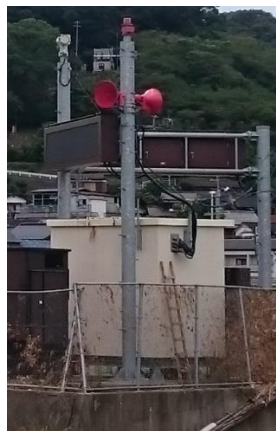
図 5 Siren & Loudspeaker of dam operator
